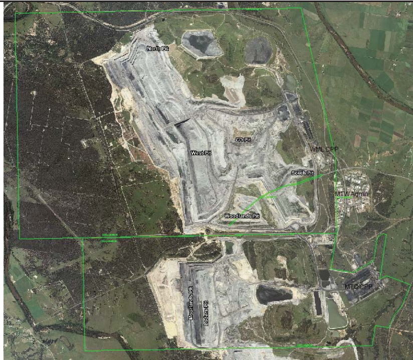
Figure 4: MTW open-cut operations
